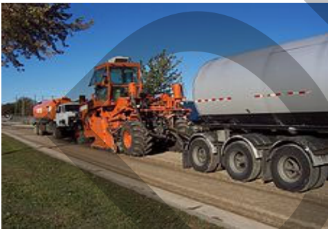
Expanded Asphalt Stabilization
