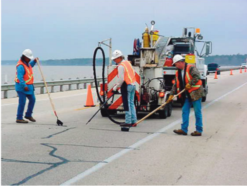
Crack Sealing
