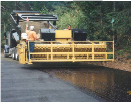
Surface Treatment (Chip Seal)
